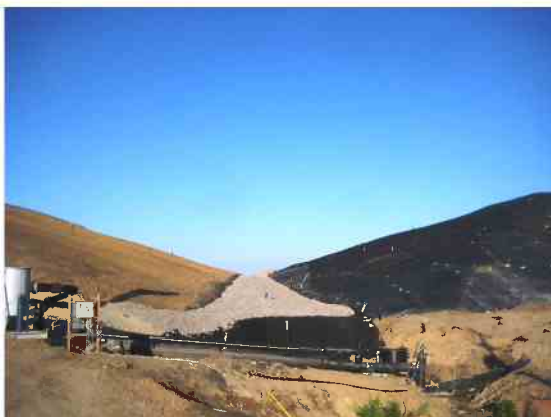
Pictured to the left is the completed isolation break.
